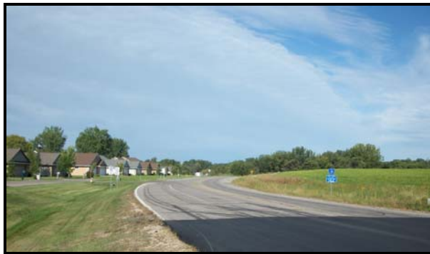
Figure 3C: Paved shoulder on paved Kandiyohi County CSAH 24
